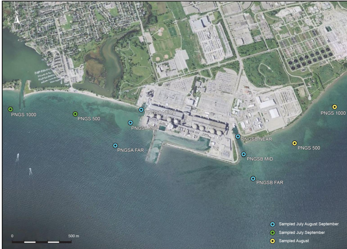
Figure H-1: Locations of the Hydrazine Sample Collections near the Pickering Nuclear Generating Station (22 July, 15 August and 10 September)
